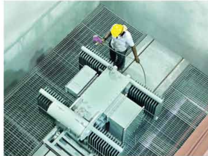
Pre delivery painting in process
